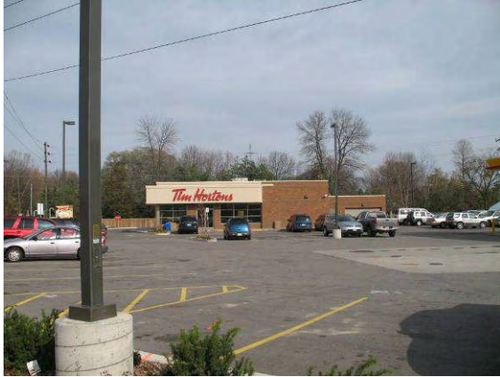
Photo 8 - 46: Southeast corner of Carlisle Road and Highway 6
